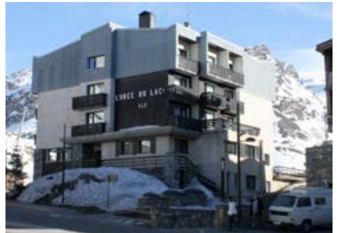
Façade principale, CAUE, 2015
